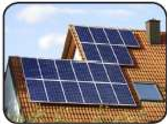
Solar panels collect energy from the Sun.
