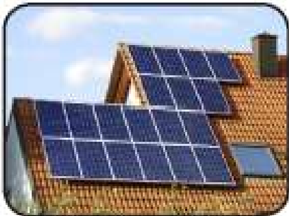
Solar panels collect energy from the Sun.
